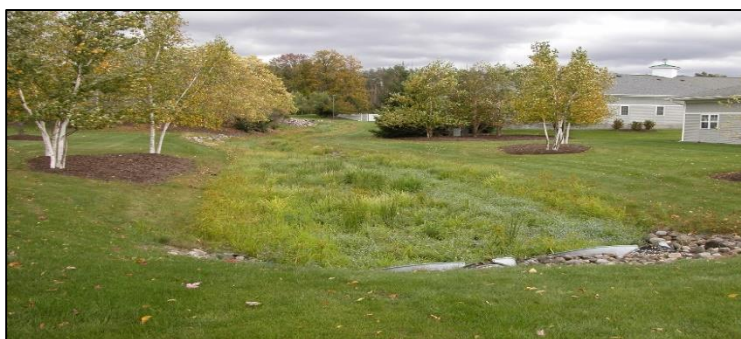
Constructed wetland for stormwater runoff provides water quality improvements, flood reduction, and wildlife benefits (Schneider 2014).
