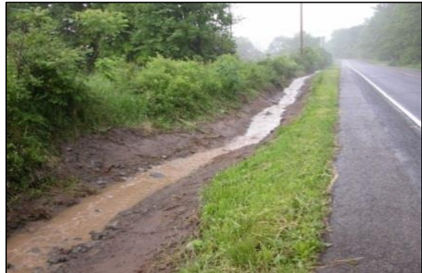
(Left) Typical method for cleaning ditches in New York. (Right) Heavy sediment load transported to stream from scraped and eroding ditch during storm event (Schneider 2014).
