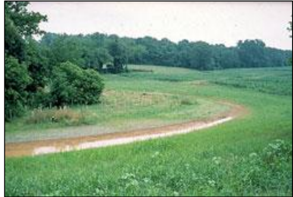
Under-road pipes (left) and level lip spreaders (right) are two strategies to diffuse stormwater discharges and reduce concentrated ditch outflows (Bloser 2014; Sweeney 2014).
