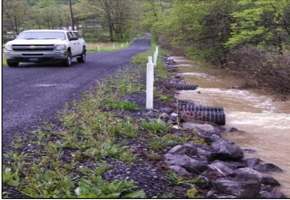
Under-road pipes (left) and level lip spreaders (right) are two strategies to diffuse stormwater discharges and reduce concentrated ditch outflows (Bloser 2014; Sweeney 2014).
