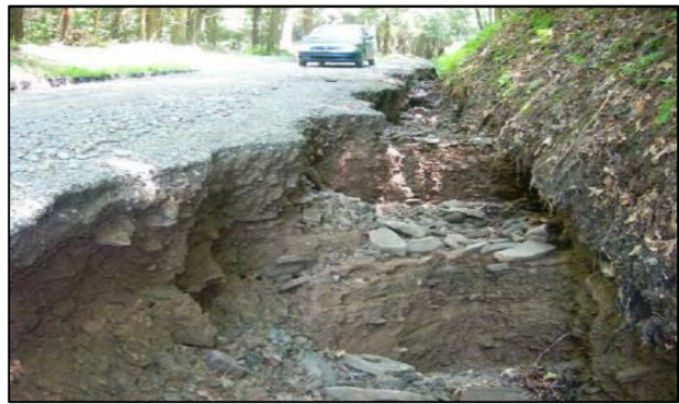
(Left) Deeply scraped, V-shaped ditch with exposed substrates (Schneider 2014). (Right) Erosion and undercutting of road surface due to erosive flows in ditch (Bloser 2014).
