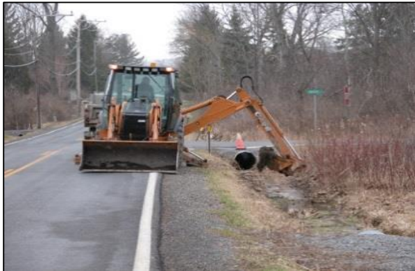
(Left) Typical method for cleaning ditches in New York. (Right) Heavy sediment load transported to stream from scraped and eroding ditch during storm event (Schneider 2014).
