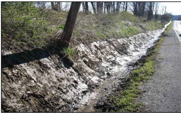
(Left) Deeply scraped, V-shaped ditch with exposed substrates (Schneider 2014). (Right) Erosion and undercutting of road surface due to erosive flows in ditch (Bloser 2014).
