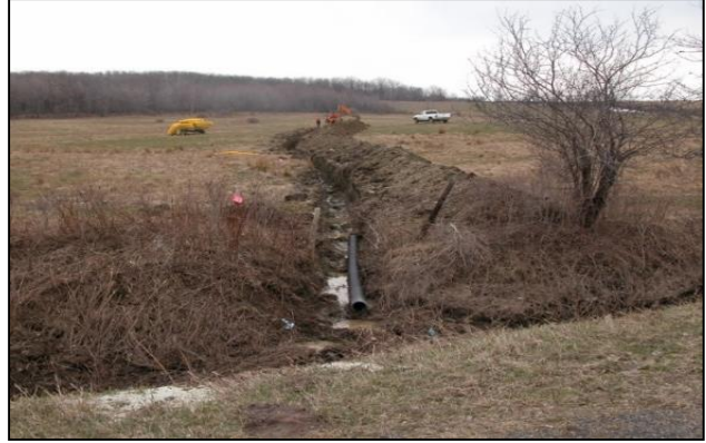
(Left) Exposed rock and gravel in ditch due to high velocity runoff and severe scouring. (Right) Installation of tile drain in farm field with outflow location in the roadside ditch (Schneider 2014).
