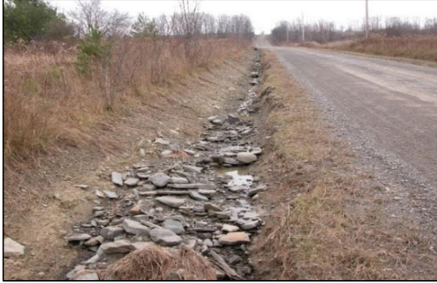
(Left) Exposed rock and gravel in ditch due to high velocity runoff and severe scouring. (Right) Installation of tile drain in farm field with outflow location in the roadside ditch (Schneider 2014).
