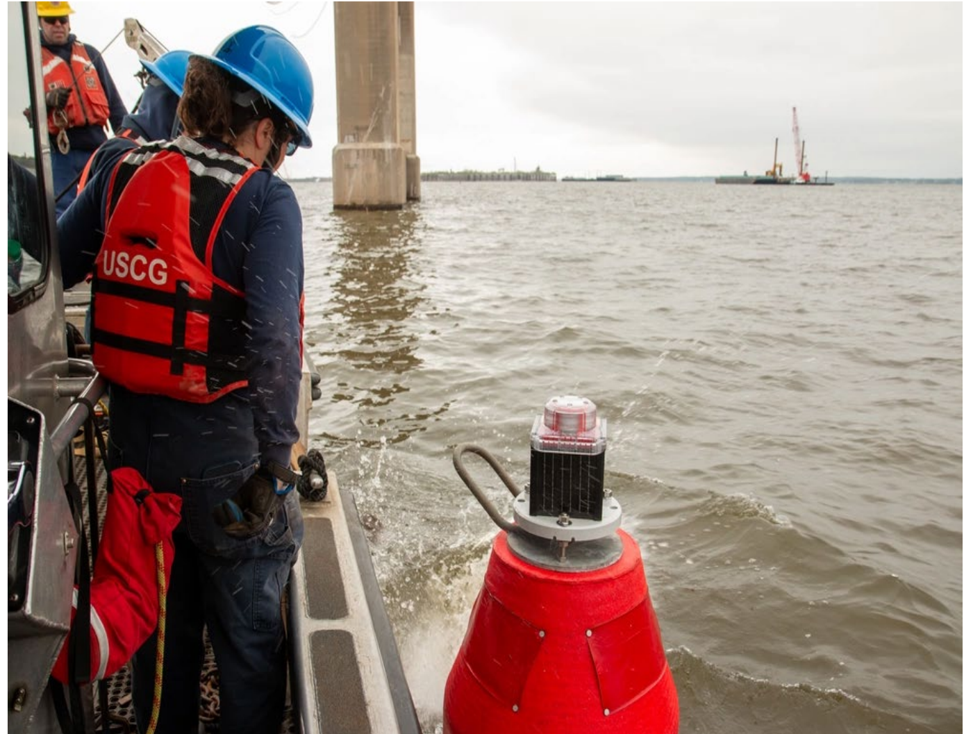
Placing buoys in preparation for the temporary channel opening
