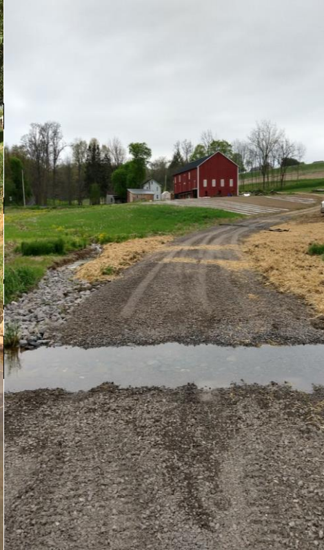
Cattle and Equipment Crossings
